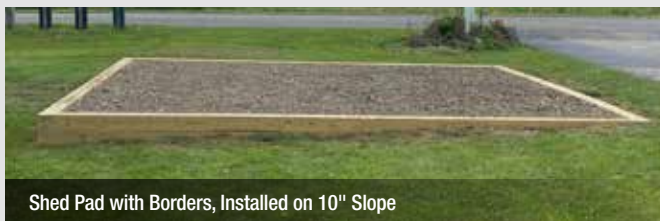
Shed Pad with Borders as Retaining Wall
