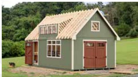
Roof rafters installed
