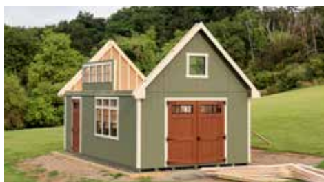
Gables set in place
