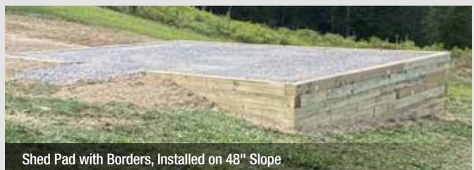
Shed Pad with Borders as Retaining Wall
